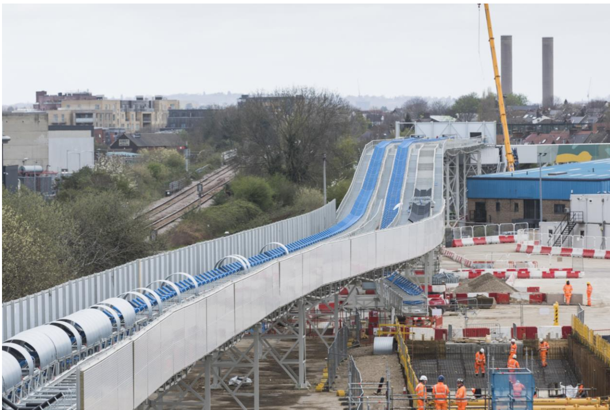
Figure 8 Atlas Road site, High Speed 2 Project, showing the spoil conveyor system.
