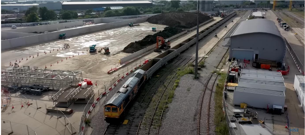
Figure 9 Willesden Euro Terminal where excavated material is received from the conveyor system and stored prior to being loaded onto trains.
