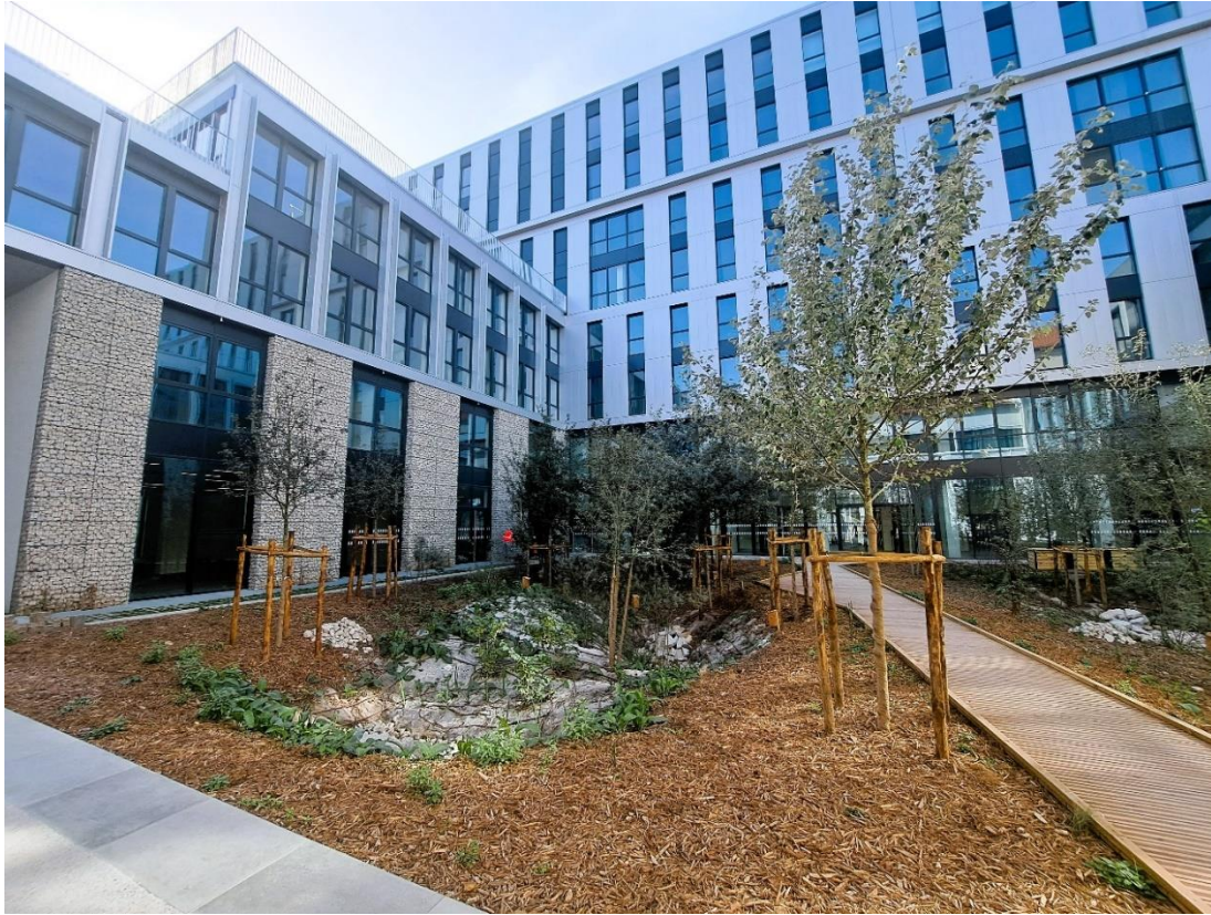
Figure 33 One of the accommodation buildings for the athletes – showing recycled concrete used in the façade of building and the gardens, recycled wood in walkways, and the overall water sensitive design of garden areas, providing green spaces and habitat for wildlife (e.g., bat boxes).
