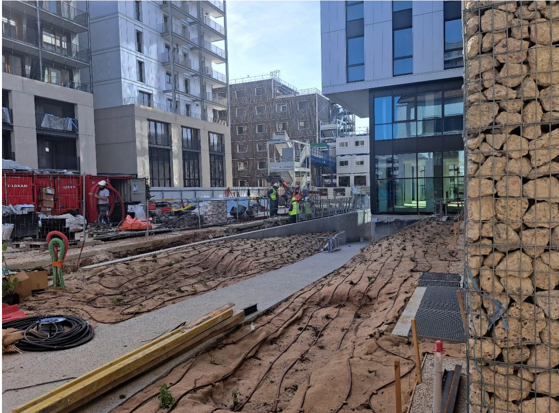
Figure 35 View of garden area which is under construction, including the extensive irrigation system to support watering with treated wastewater year-round.
