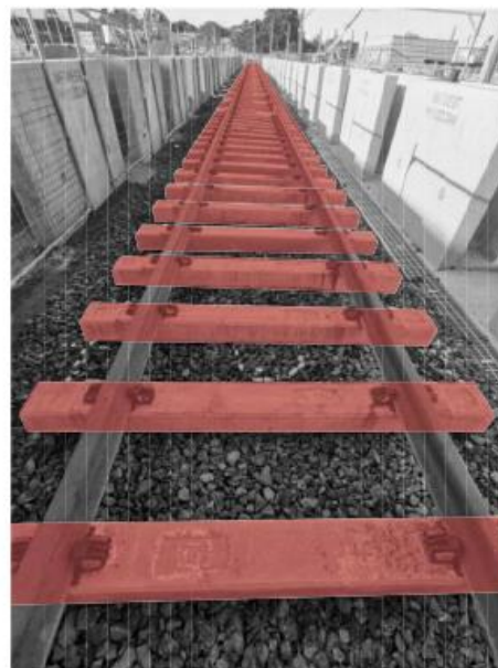
Geopolymer concrete sleepers with 60% lower carbon footprint than standard concrete sleepers at a Sydney Metro maintenance facility.
