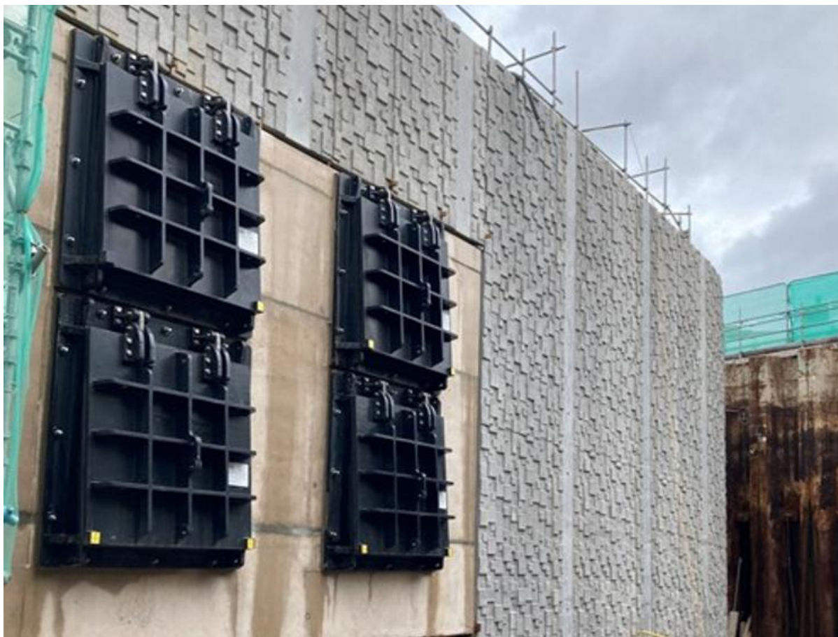
Figure 14 Intertidal River wall using a geometric design to provide ‘shelving’ to retain moisture and promote colonisation (Tideway London, 2023)
