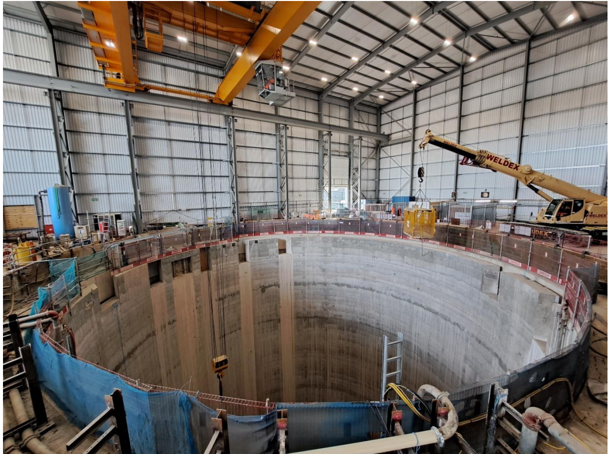
Figure 28 View into the huge shaft at Tideway East, Chambers Wharf site – 28m wide, and 60m deep.
