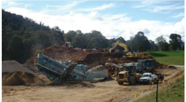
Recycling excavated material for use as a road base.
