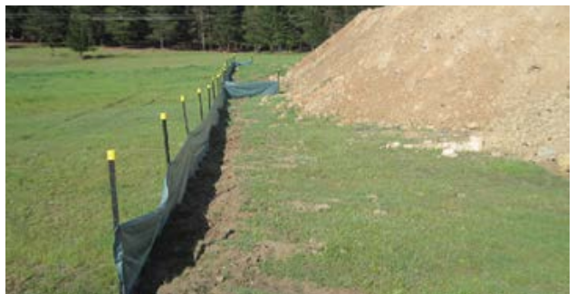
Sediment fence downslope of spoil stockpile.
