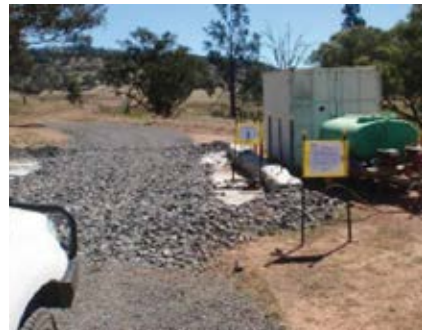
Temporary vehicle wash bay facility for preventing the spread of invasive weeds and diseases.
