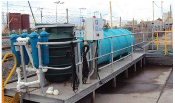
Triple interceptor wastewater treatment system.
