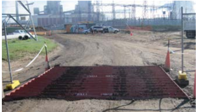
Site access stabilised with cattle grid to prevent tracking of sediments offsite.
