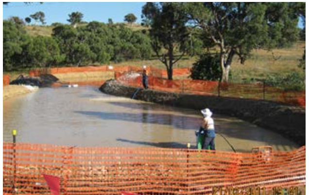
Flocculation of a sediment basin.
