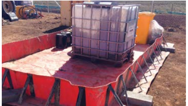
Temporary bund for storage of hazardous liquids.
