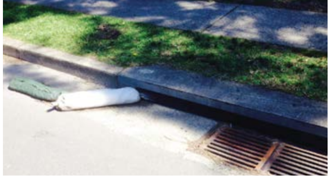
Protection of a stormwater drain using silt socks.
