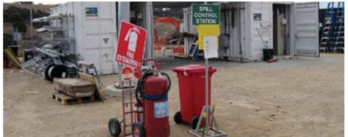
Spill response kit located at a designated spill control station.
