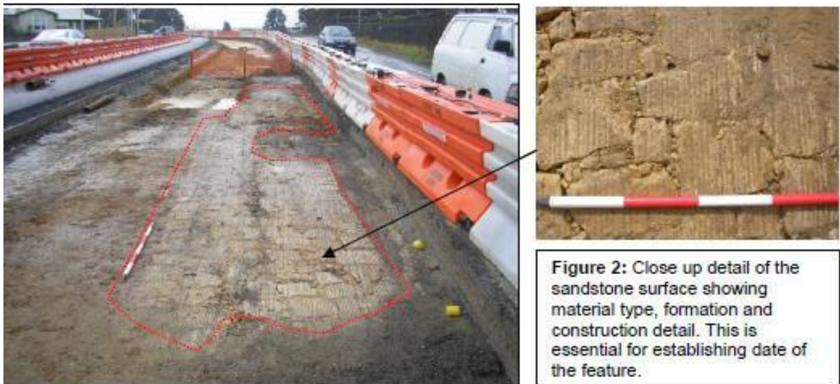
Figure 1: Telford road uncovered on the Great Western Highway (Leura) in 2008 (RMS, 2015).
