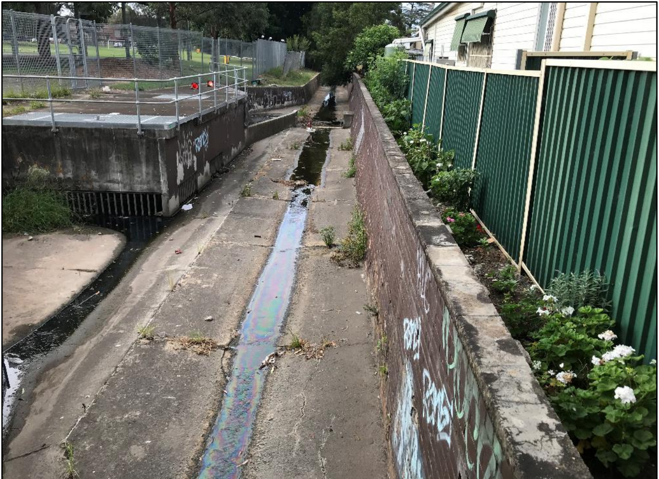
Photograph 1. Condition observed from sampling location of WP1 during the monitoring event – 10 March.
