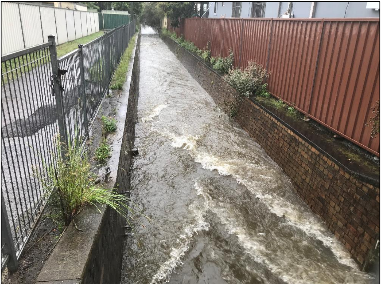
Photograph 4. Condition observed from sampling location of WP2 during the monitoring event – 20 March.
