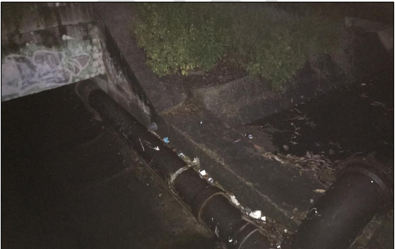
Photograph 4. No water flow observed from the discharge point which is located within the rail corridor and immediately upstream / south from WP2 during the monitoring event – 5 May.
