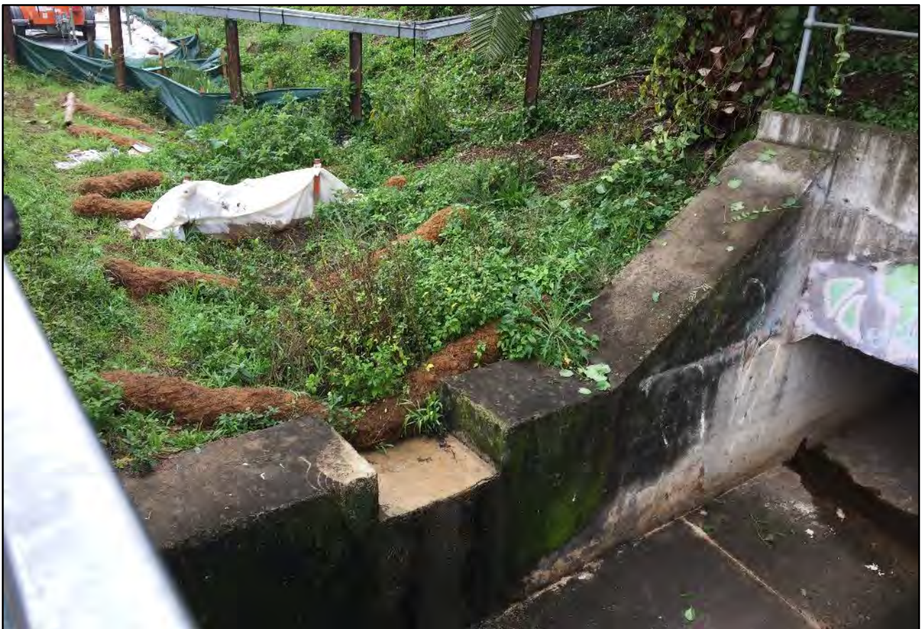
Photograph 4. No stormwater in-flow observed from the discharge point WP2-DP1 which is located within the rail corridor and immediately upstream / south from WP2 during the monitoring event – 1 July.
