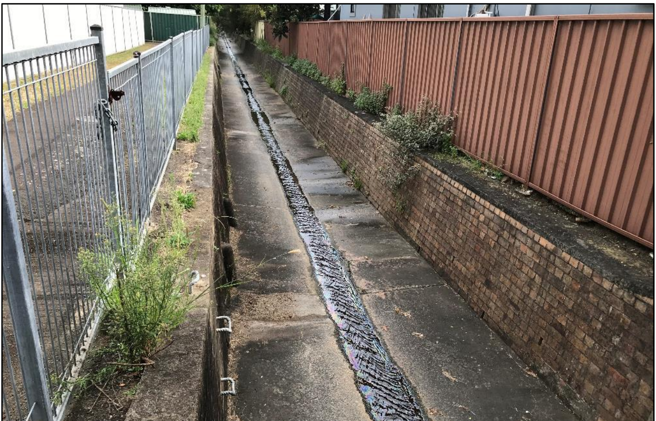
Photograph 2. Condition observed from sampling location of WP2 during the monitoring event – 10 March.
