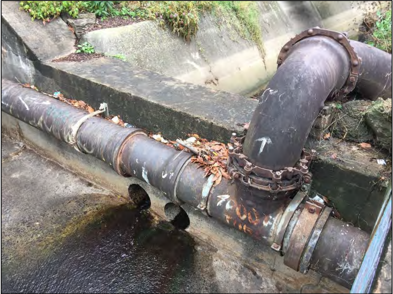
Photograph 5. Stormwater in-flow observed from the discharge point WP2-DP2 which is located within the rail corridor and immediately upstream / south from WP2 during the monitoring event – 1 July.
