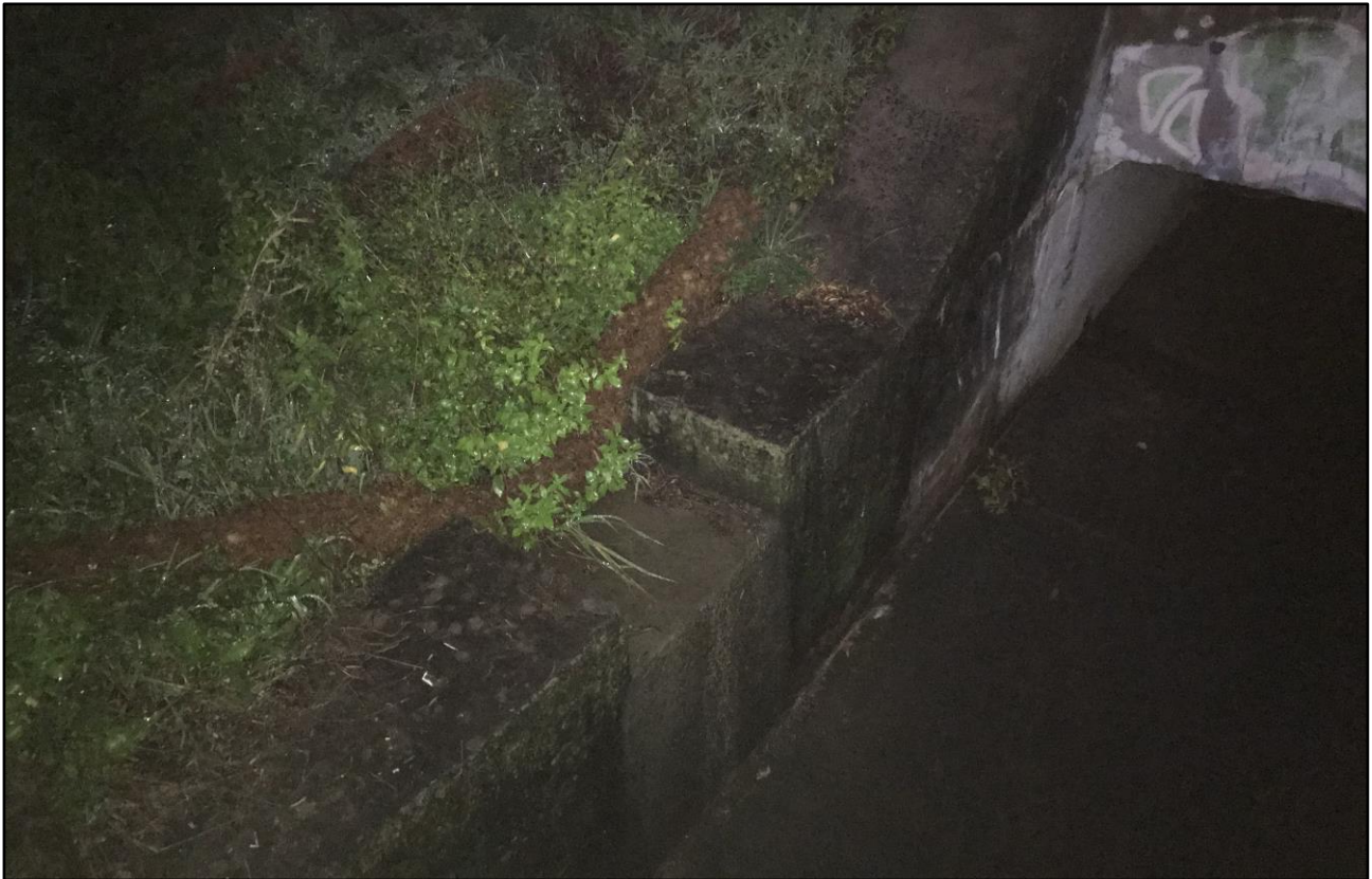
Photograph 3. No water flow observed from the discharge (the one connecting the construction site and the unnamed channel) which is located within the rail corridor and immediately upstream / south from WP2 during the monitoring event – 5 May.
