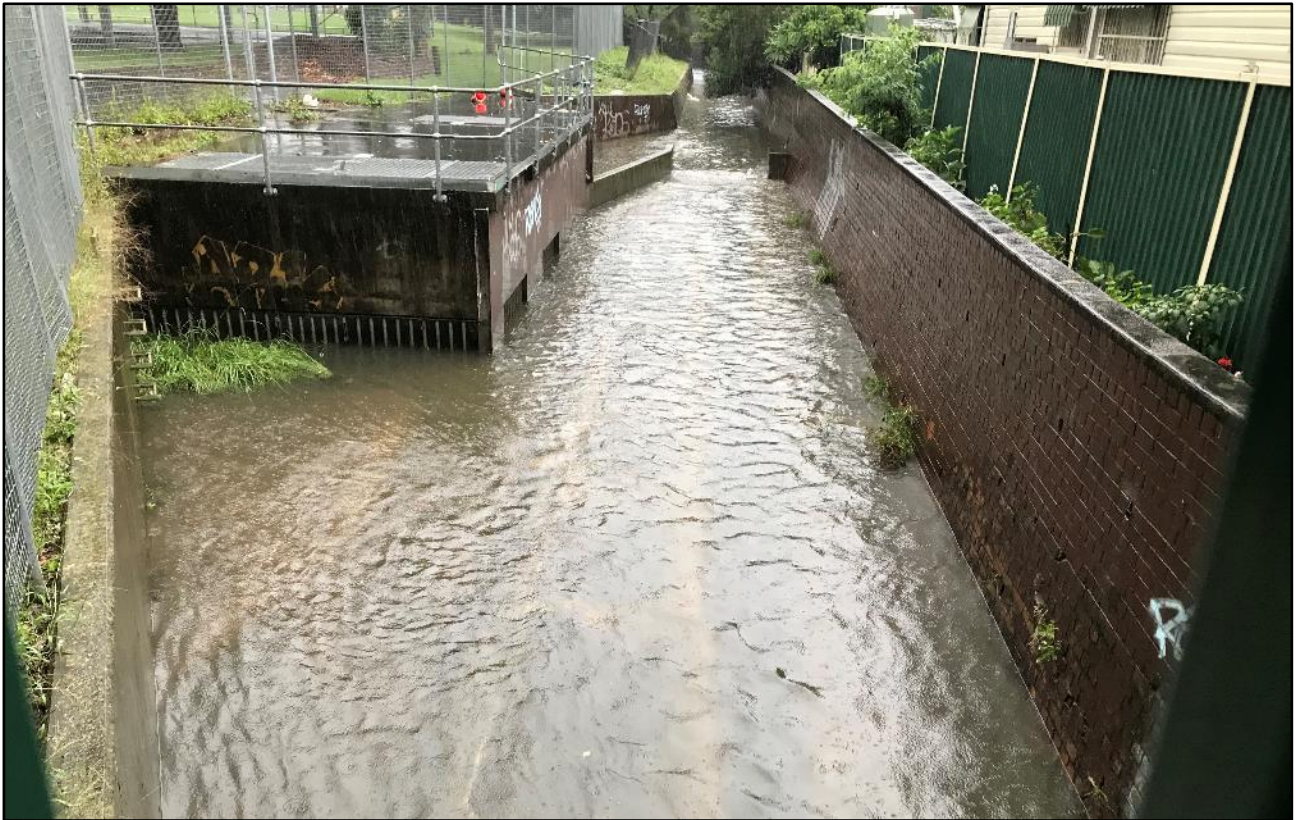
Photograph 3. Condition observed from sampling location of WP1 during the monitoring event – 20 March.
