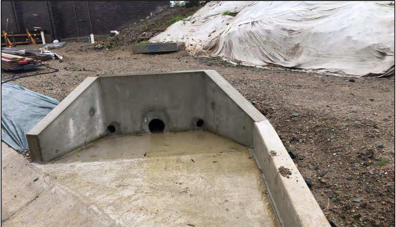
**Photograph 13.** Downstream discharge point (the middle conduit of the Head Wall 1) of the surface water collected by the Platform 1 drainage system. It is noted that the two smaller diameter conduits on the sides are not connected to any drainage system and only functioned as weepholes. Date: 5 October 2022.
