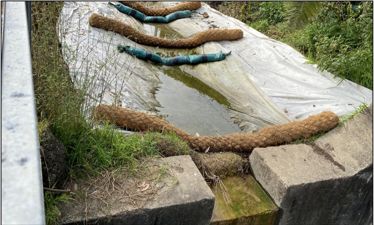
**Photograph 5.** Current condition and sediment / erosion control of the downstream discharge point WP2-DP1 which were located within the rail corridor and immediately upstream / south from WP2 during the monitoring event – 25 August 2022.
