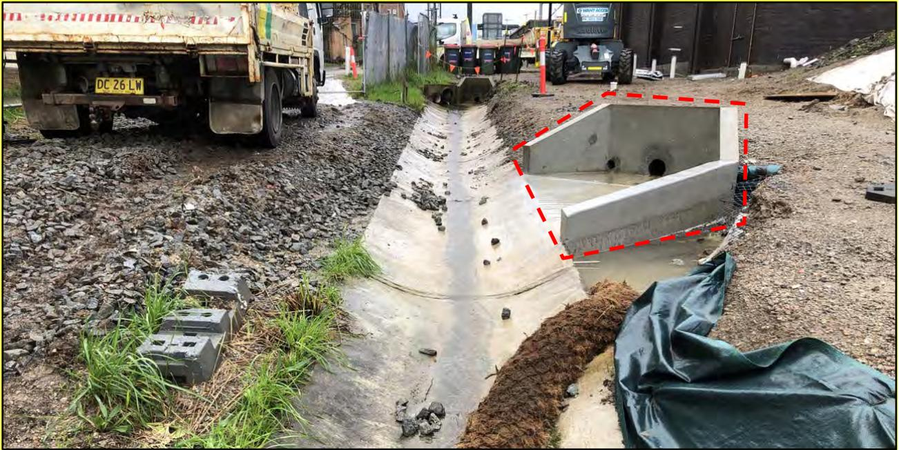
**Photograph 7.** Identified flow contribution to WP2-DP1: platform drainage – stormwater and it was mixed with urban runoff inflow once entering into the concrete lined swale. Date: 21 July 2022.
