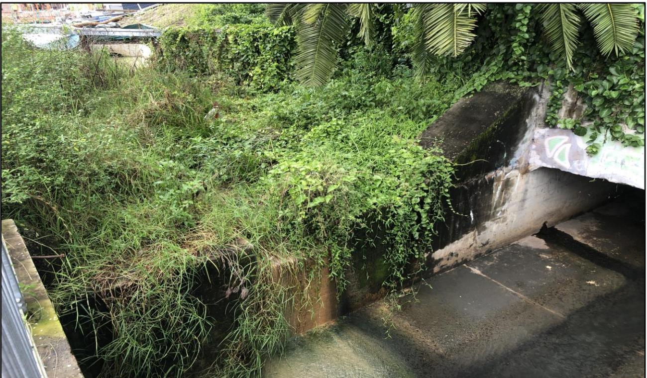
**Photograph 4.** Low level of flow contribution was observed from downstream eastern discharge point WP2-DP1. Date: 24 May 2022.
