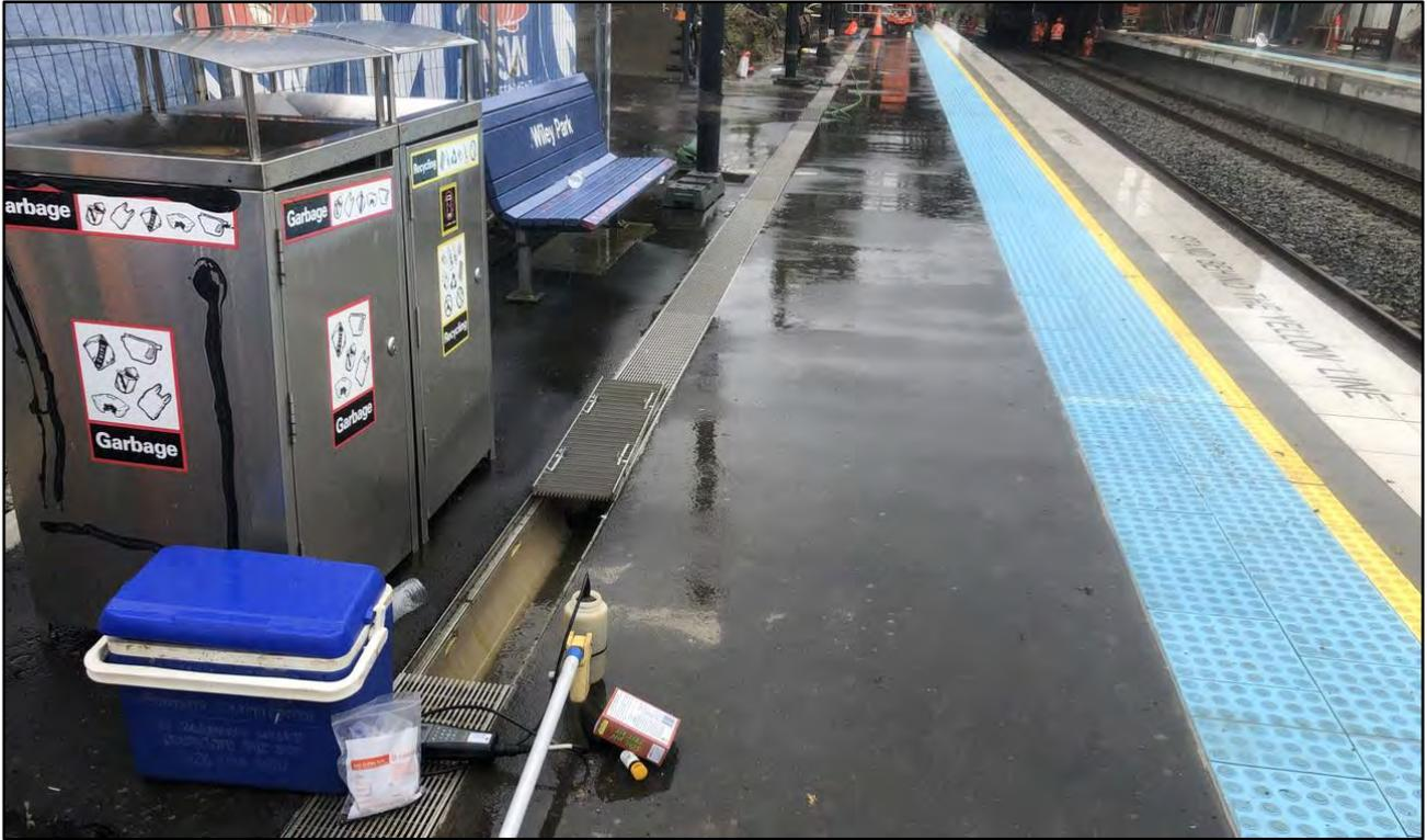
**Photograph 7.** Aco drain check – tap water test. Date: 5 October 2022.
