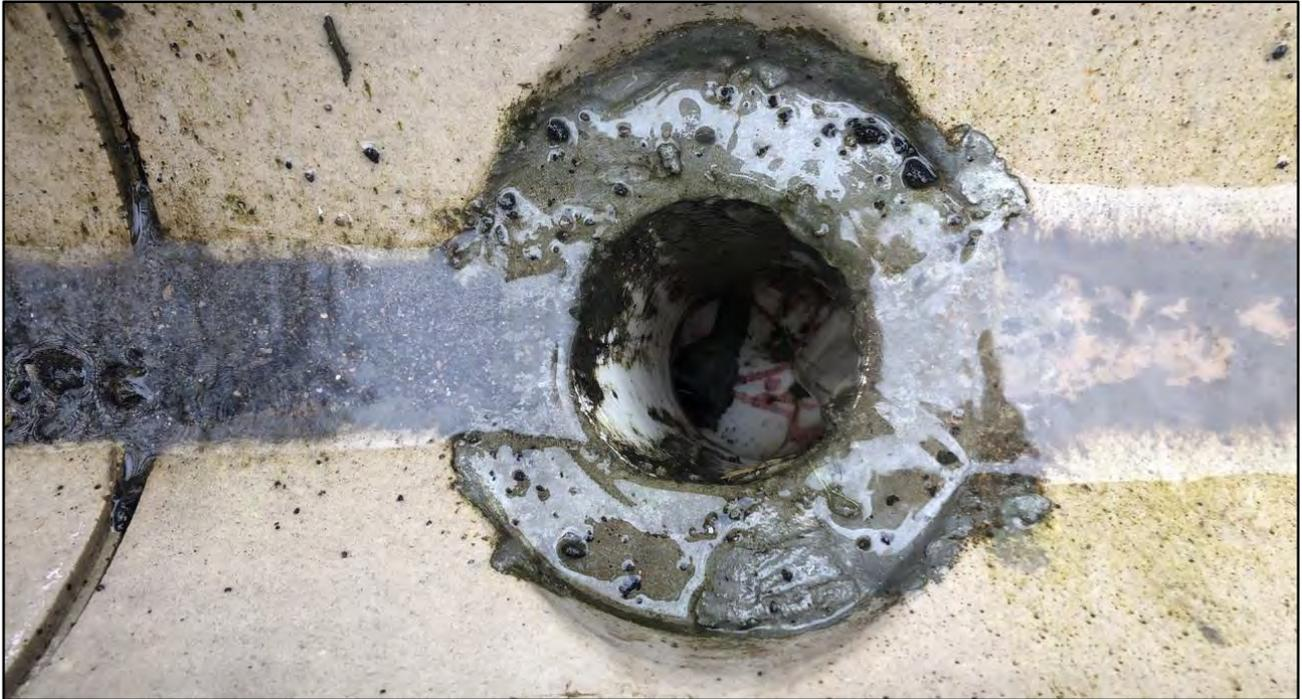
**Photograph 11.** Aco drain check – additional observation – drainage point. Date: 5 October 2022.
