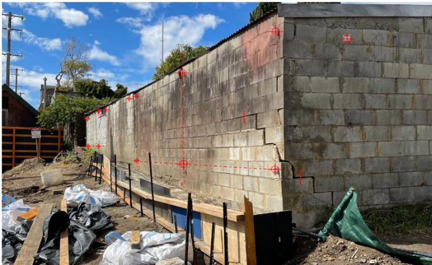
— Denotes location and orientation for crack gauge (pack out and bond to blockwork) (3 locations)
