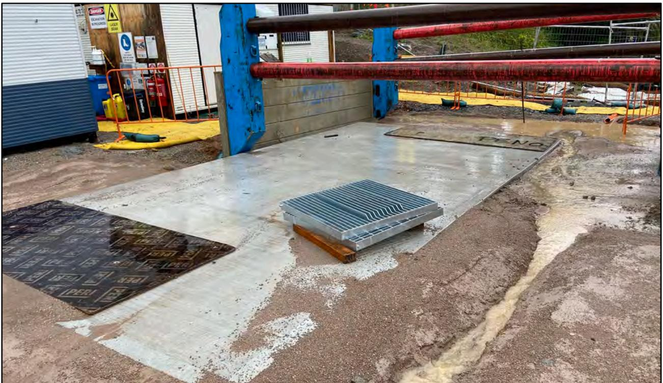
**Photograph 8.** Identified flow contribution to WP2-DP1: temporary surface water erosion and sediment control trenches and area surrounding constructed OSD tank. Date: 4 July 2022.
