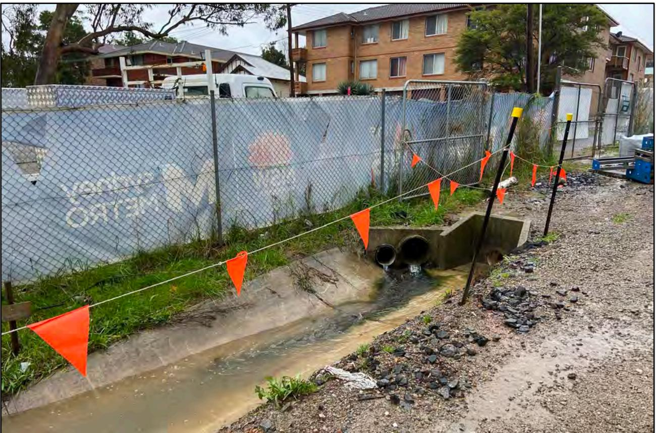
**Photograph 6.** Identified flow contribution to WP2-DP1: urban runoff drainage – stormwater. Date: 4 July 2022.
