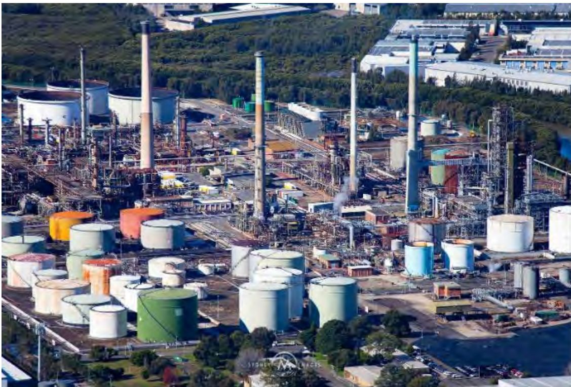
Plate 2 Former Clyde Refinery infrastructure prior to demolition
