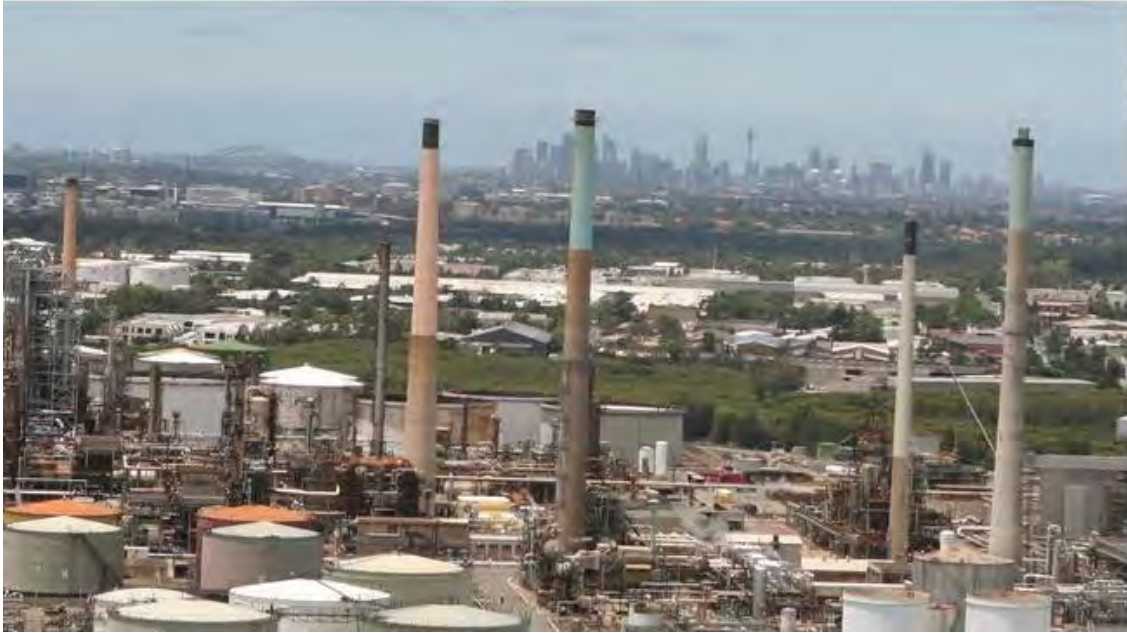
Plate 1 Former Clyde Refinery chimney stacks prior to demolition
