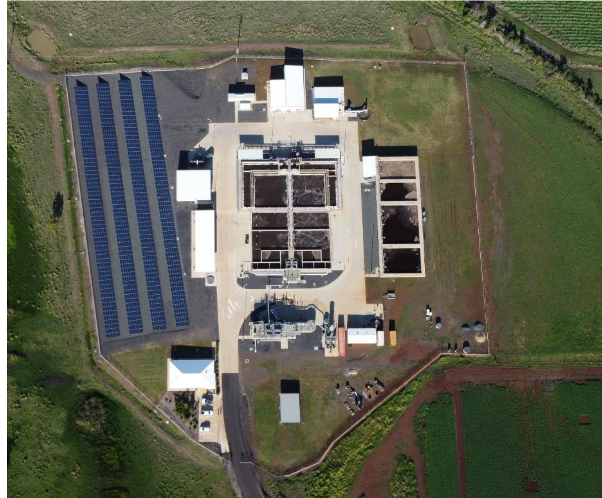
Rubyanna wastewater treatment plant
