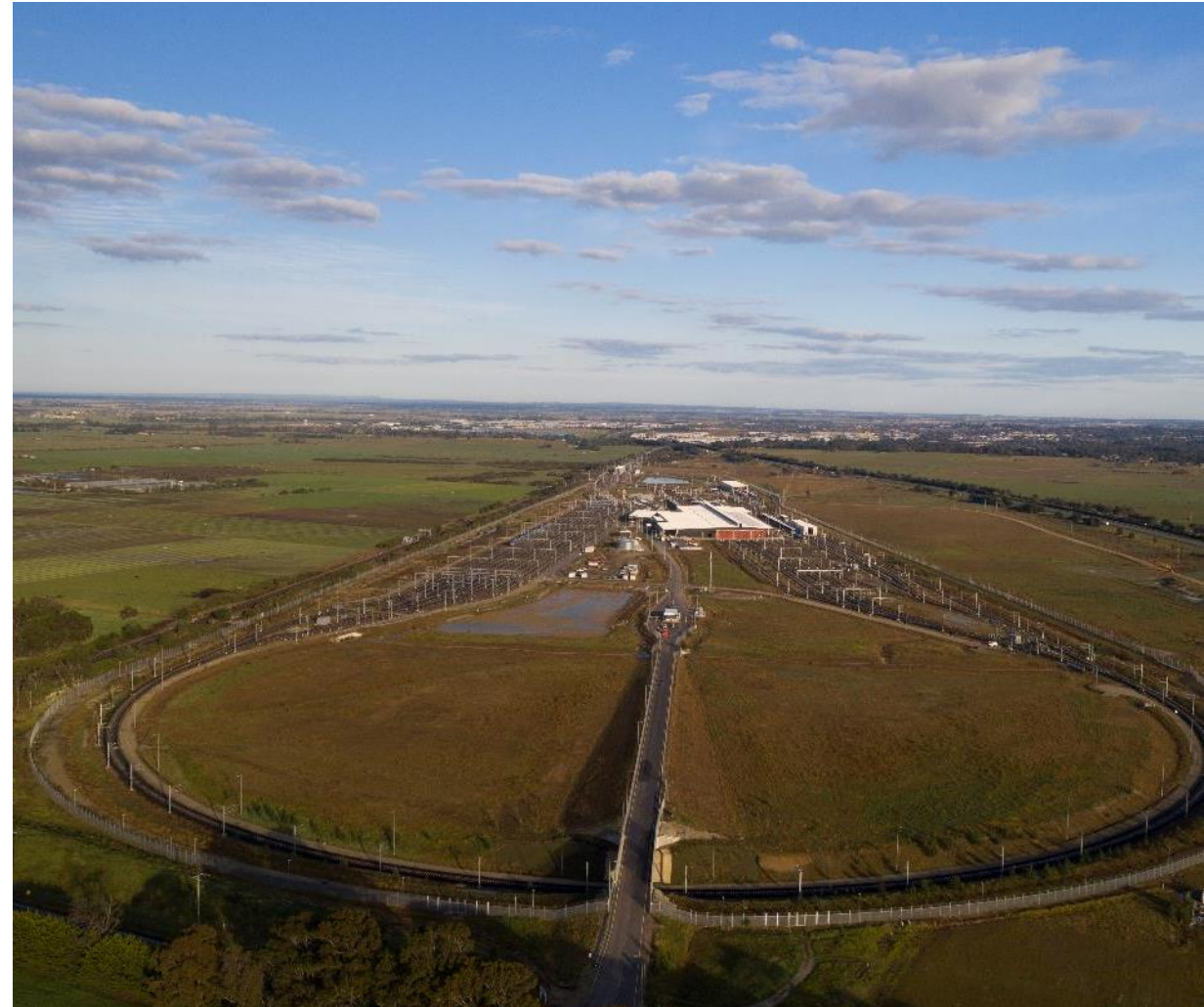
HCMT Pakenham East Maintenance Facility, Australia's largest rollingstock depot
