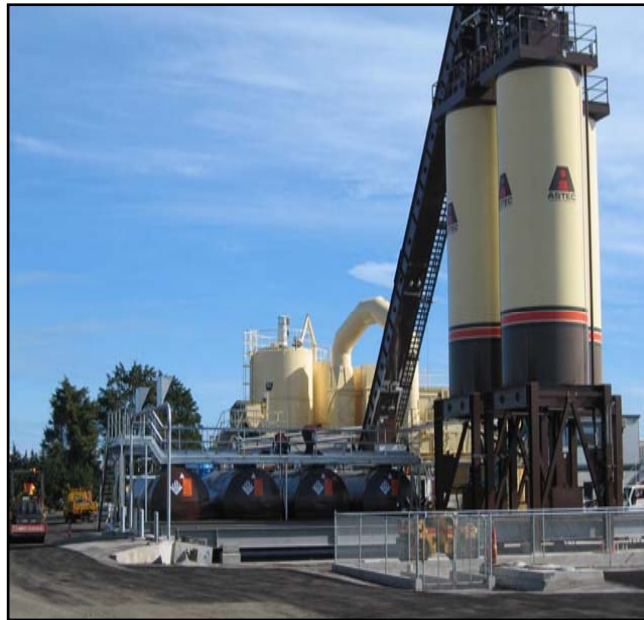
Transportation – Road Asphalt Plant
